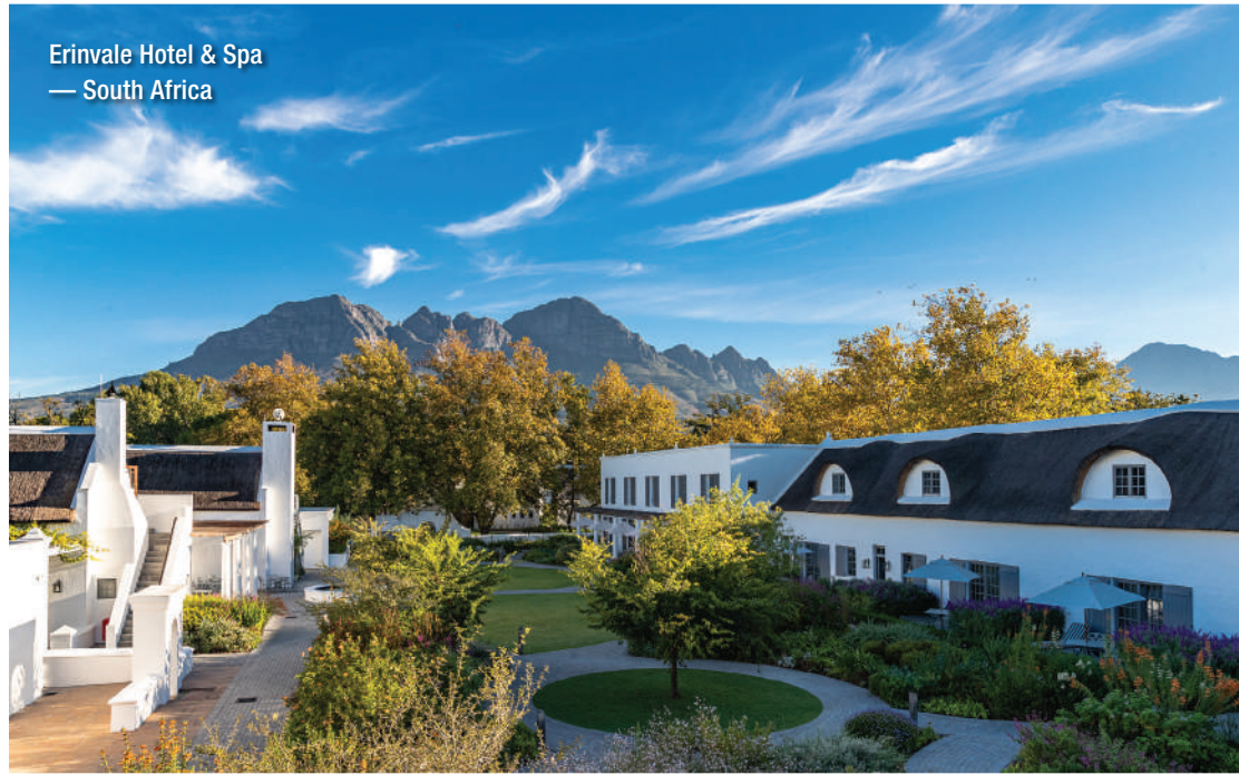
PHOTO COURTESY OF ERINVALLE HOTEL & SPA
